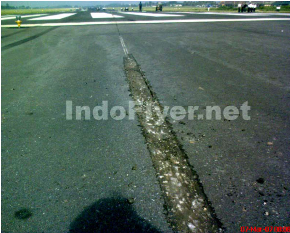
Nose gear rim ground contact ( indoflyer.net )
