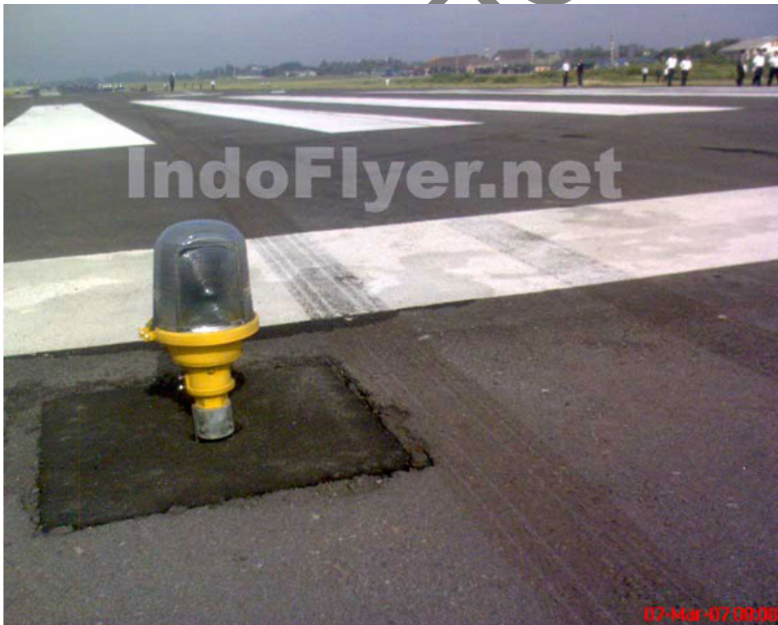
Heavy Braking Marks ( indoflyer.net )
